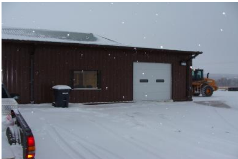
East Side Maintenance Bay
